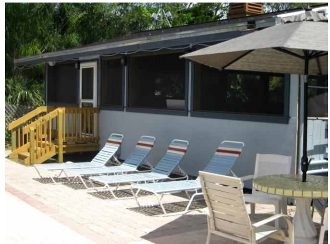
Pavilion Front Repair Completed
